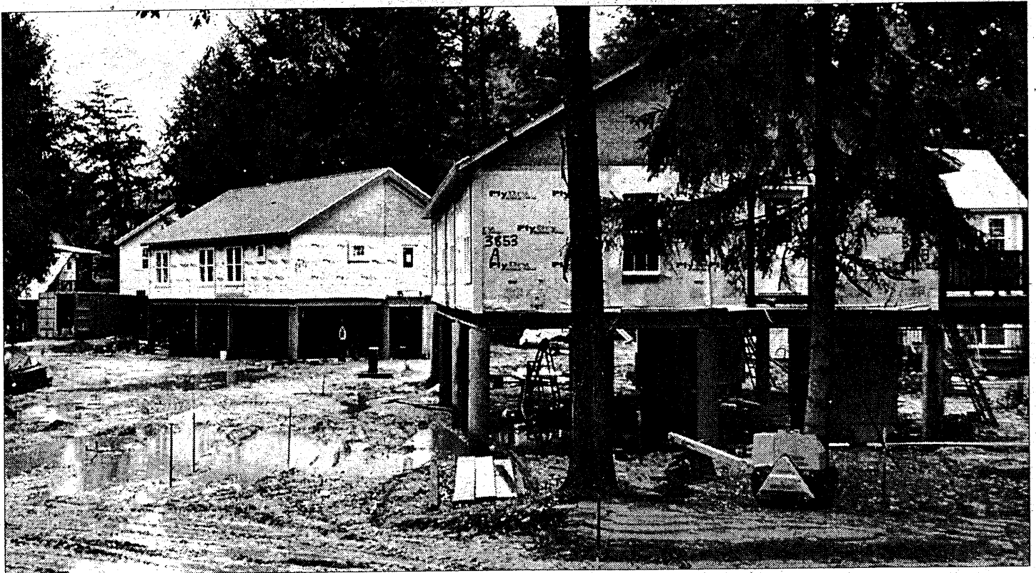
The Pine Woods affordable housing complex off Route 102 in Stockbridge continues to take shape. Though portions of the work site were reduced to a muddy and water-logged state due to the recent round of rainy weather, the development is on track for completion later this year.
